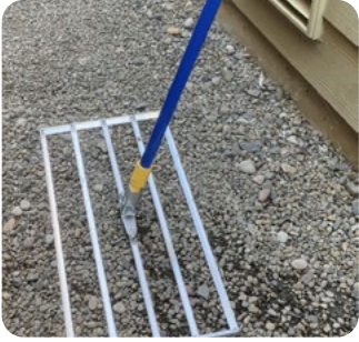
Leveling aggregate
