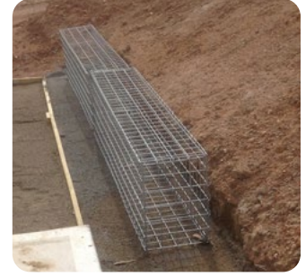
Gabion wall install
