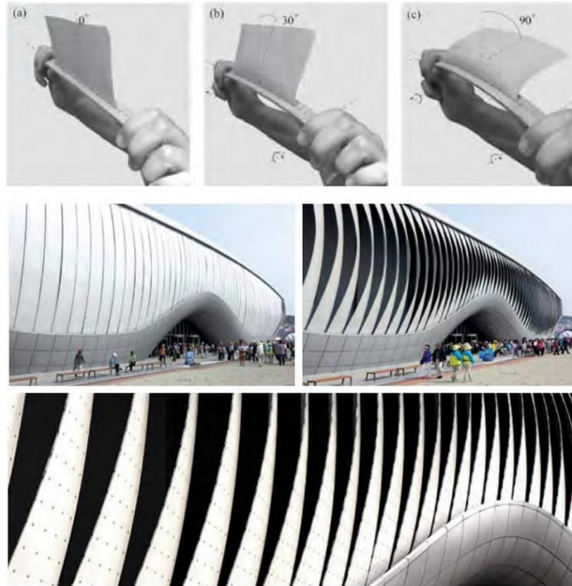
Fig.22-24: Kinematic facade of the Thematic Pavilion EXPO 2012 in Yeosu, South-Korea. Architects: soma-architecture, Vienna; Engineer for Kinetic Facade: Knippers Helbig, Stuttgart, New York.
