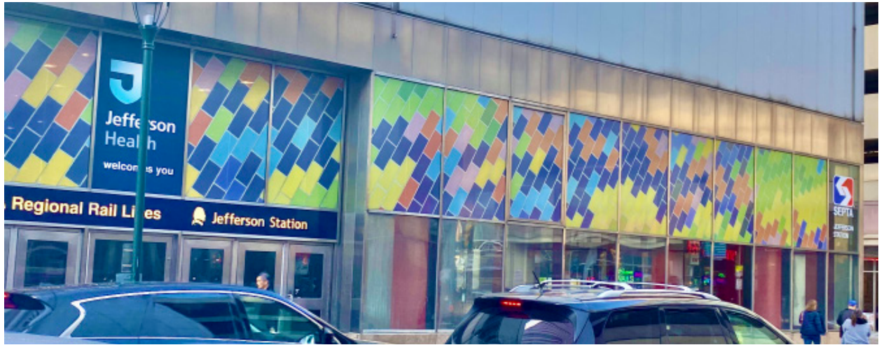
Jefferson Station, Center City section of Philadelphia.
